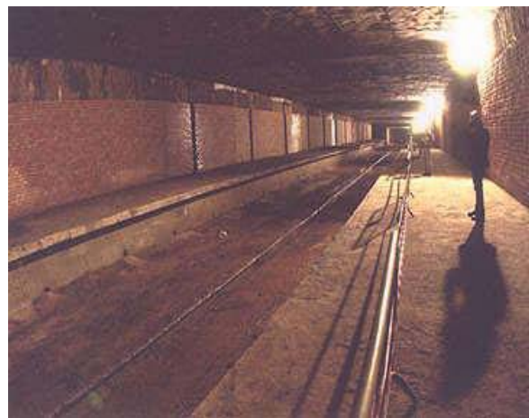
Figure 2 annex 3.2: Sevilla Metro tunnel
